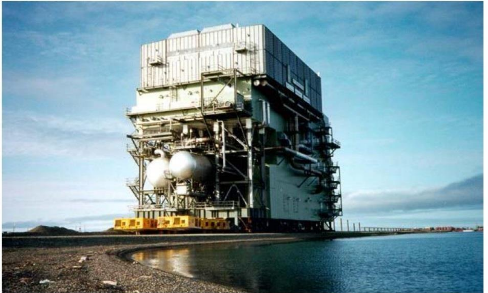
Land Transportation for Complete Modules on SPMT Trailers
